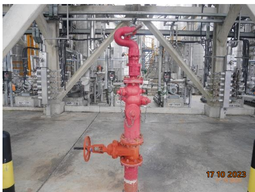
Fire Water Monitor with Foam Induction
