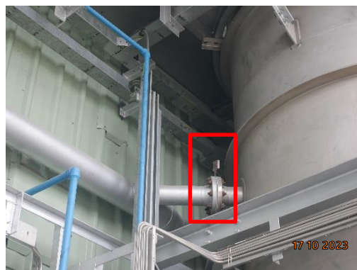
Rupture Disc
