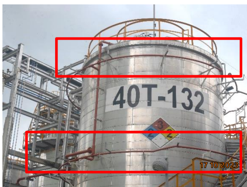
Automatic Water Sprinkler System
